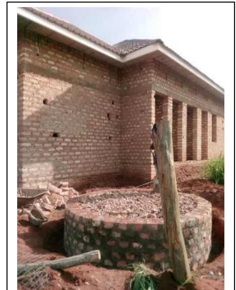
The foundation for the water tank outside Rehema's new training centre
