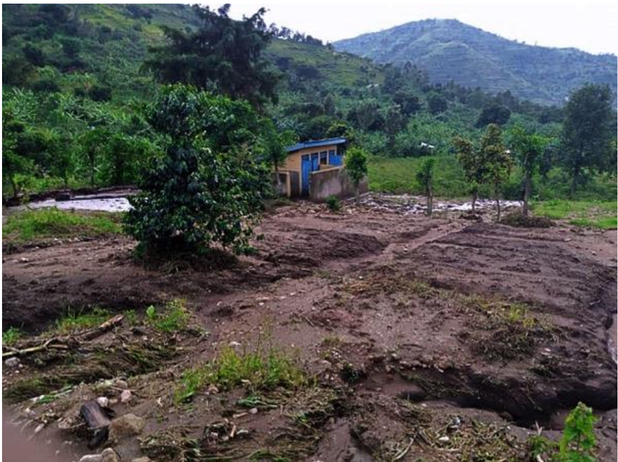
Isule Primary school: The classrooms were all swept away, leaving only the toilet
