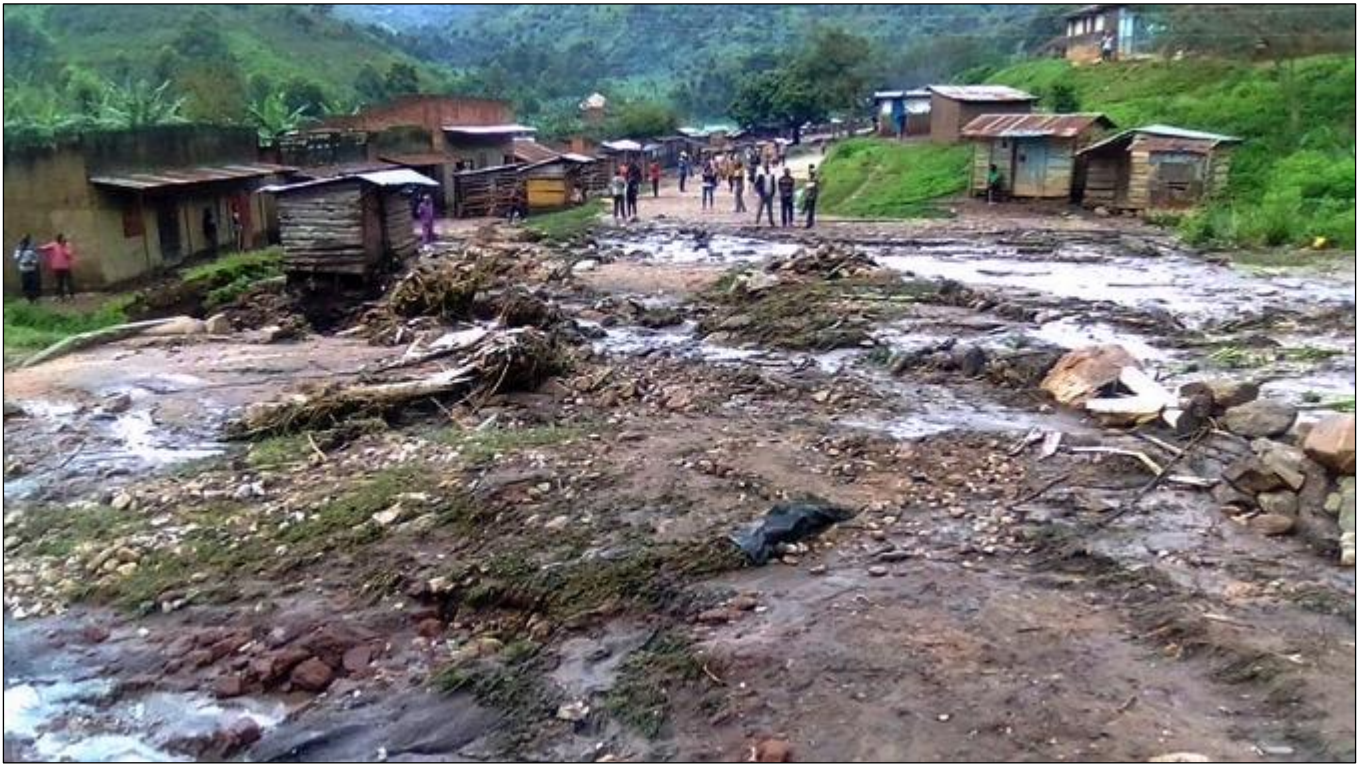
A small trading centre where people go to buy food and items for daily use was swept away and 34 houses were destroyed
