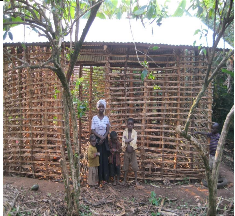
After receiving the iron sheets, a new house was set up. The new iron sheets were roofed on a new house.
