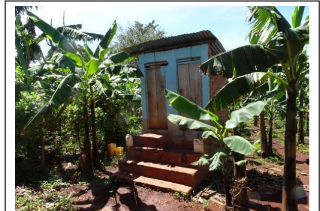
This robust compost toilet stands at the edge of Andrew and Irene's banana plantation. Faeces and urine are both used to fertilise the farm.
