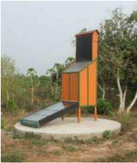
A large solar drier at Baobab Children Foundation, Cape Coast, Ghana. Notice the concrete base. The entire unit is on wheels so that it can be rotated, such that the solar collector always directly faces the sun.
