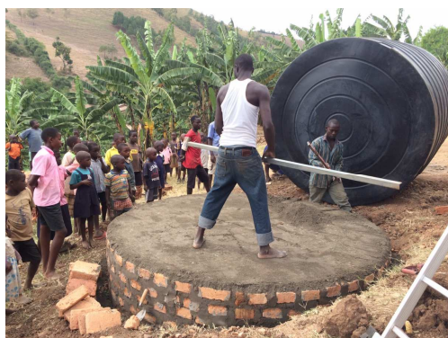
Two of these much larger rainwater tanks will hopefully be installed in Nyiruvu Village, near Arua, Uganda.
