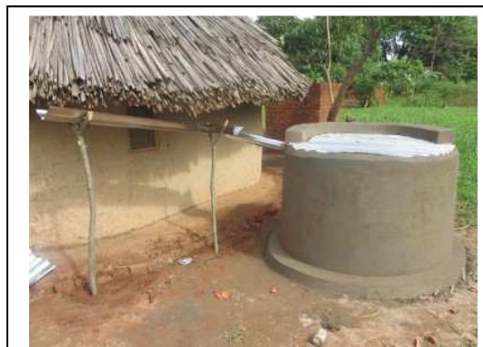
This is the sort of tank that Discover hopes to provide for 50 houses in Kirembe Village, near Kasese, Uganda.
