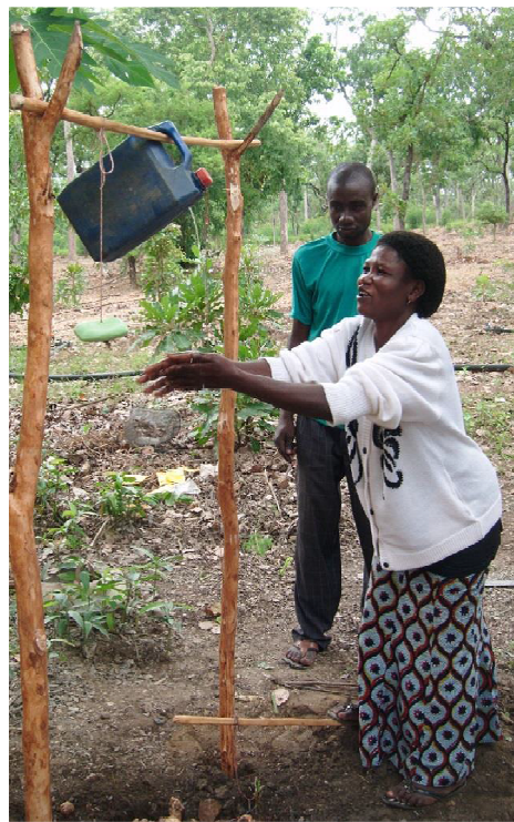
This tippy tap was constructed during a SALEM training seminar in Togo in 2014. Note the hole under the tippy-tap which is filled with stones to make a soakaway.
