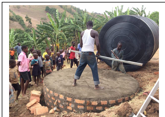
Two of these much larger rainwater tanks will hopefully be installed in Nyiruvu Village, near Arua, Uganda.
