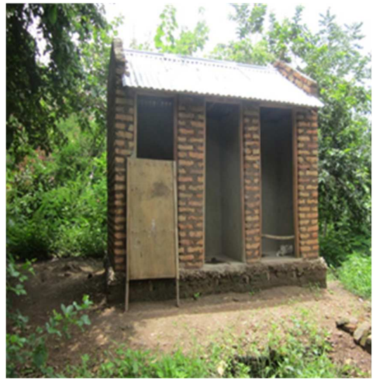
Toilet No. 2. A clean, well-built toilet, well placed, but needing a permanent door.
