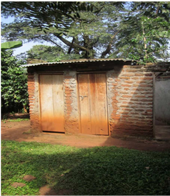
Toilet No.3 is in good condition and always used by the family. Nobody in this home has suffered even diarrhoea during the past two years.
