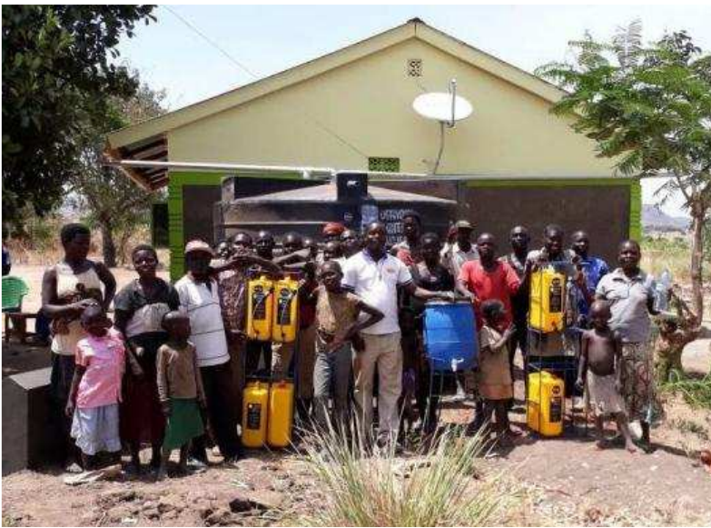
A water tank in Nyirivu Village is finally in place, on a strong foundation, and with the associated guttering and pipework. The villagers are thrilled, especially those who helped with the construction
